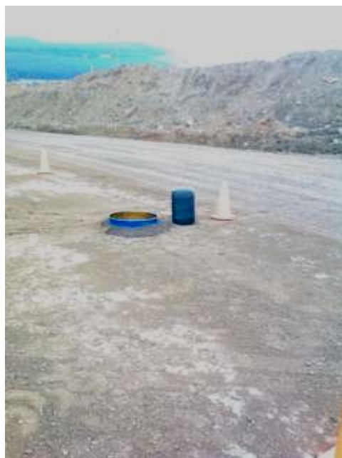
Figure 3. Wearing course is soaked before performing DCP test.
