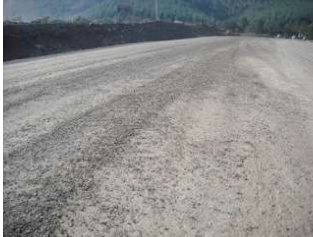
Figure 2. View of the Polymer stabilized trial section with spillage from trucks.
